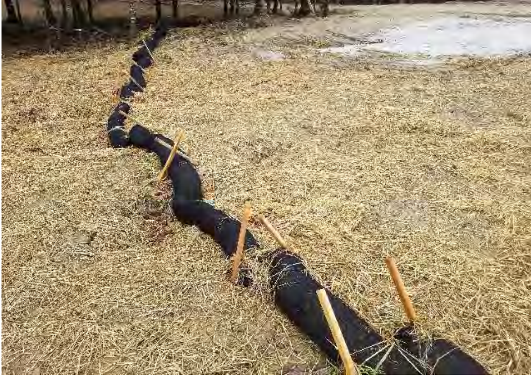
Fig 15: Erosion underneath filter sock downslope of Str. 99 at Getchell property/west side of the Bay. Ground surface in upper right corner is stable. See comments above. Viewing west. (03-30-20).
