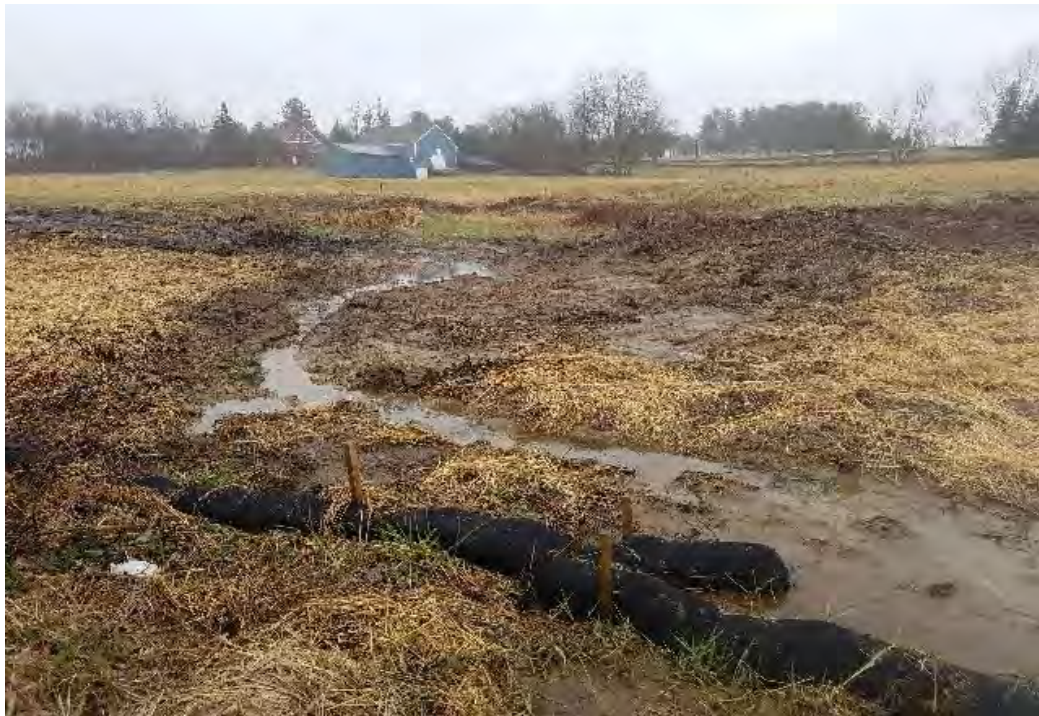
Fig 4: Erosion in wetland NW18 at Frink farm. See comments above. Viewing southeast. (03-30-20).
