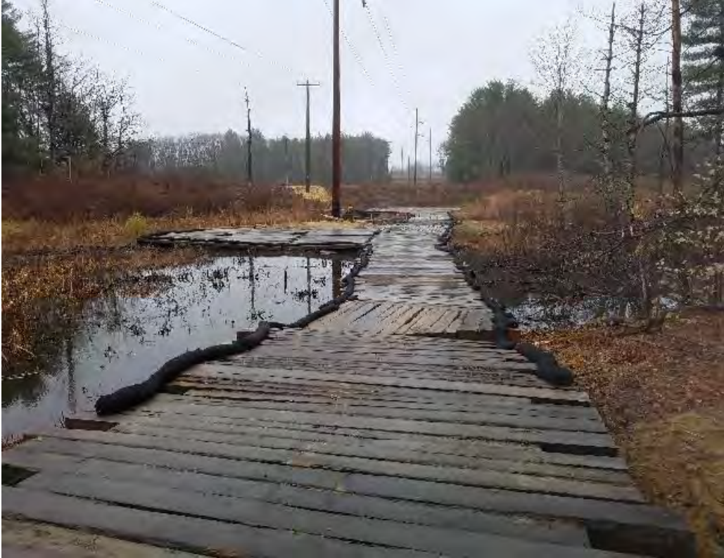
Fig 9: Access road to Str. 114, through wetland NW17. Viewing east. (03-30-20).
