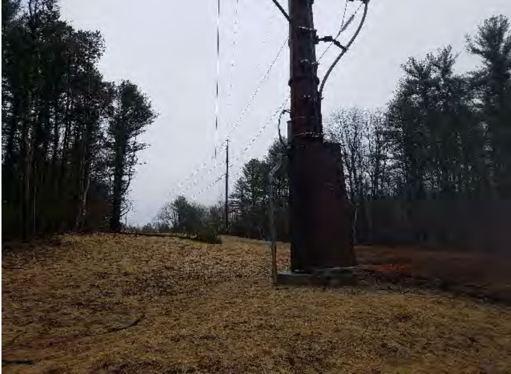
Fig 3: Str. 100 foundation. Viewing east. (03-30-20).
