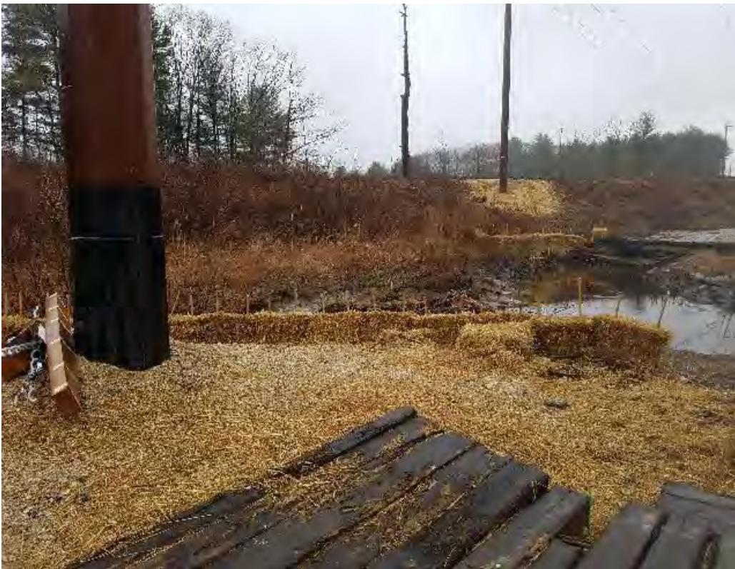
Fig 10: Strs. 114 and 3850-64 foundations. Viewing east. (03-30-20).
