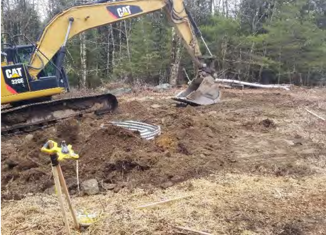
Fig 17: Crew restoring work area around Str. 76 foundation can. Viewing west. (03-30-20).
