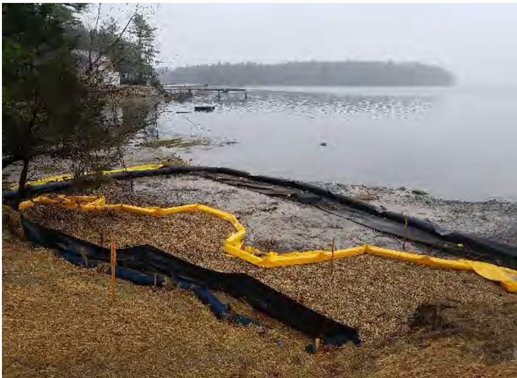
Fig 2: Turbidity curtain in intertidal zone at Gundalow landing/east side of the Bay. Viewing south. (03-30-20).
