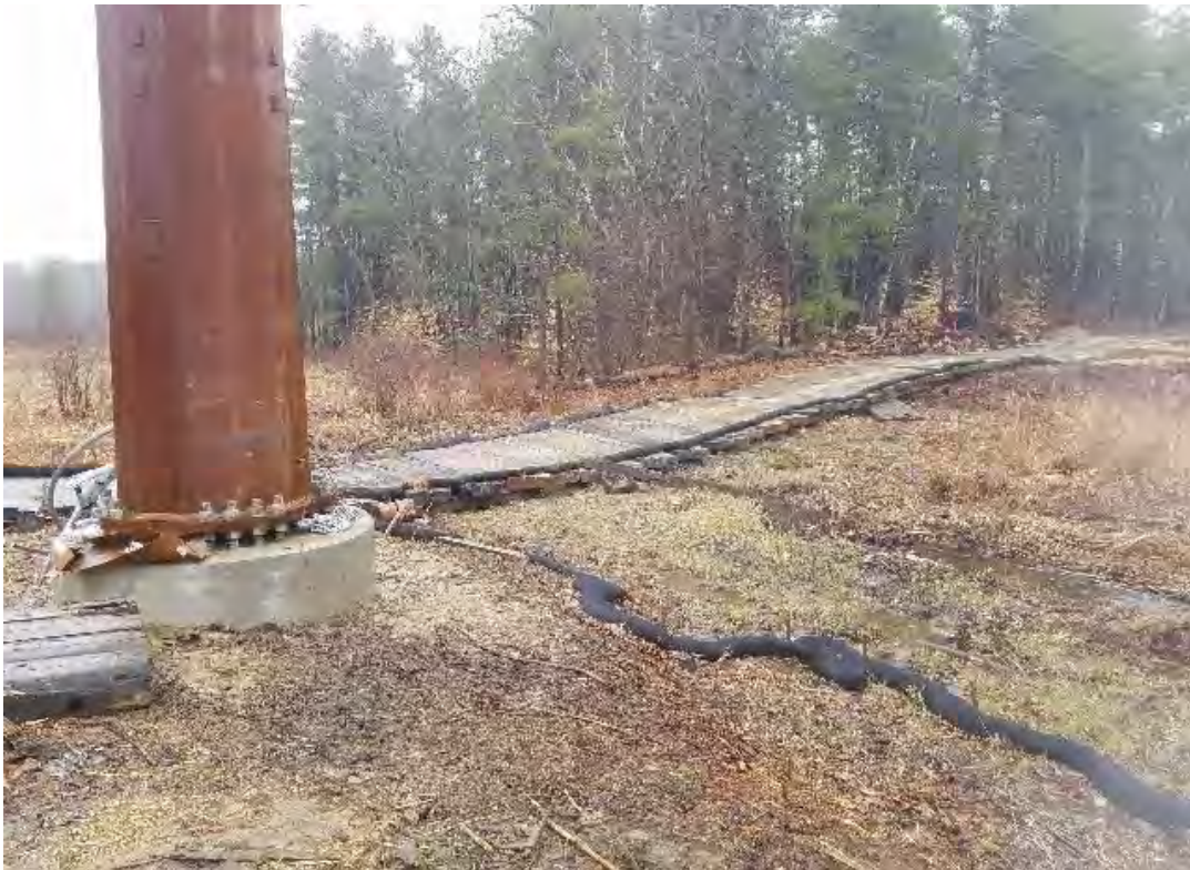
Fig 8: Str. 112 foundation. Viewing east. (03-30-20).
